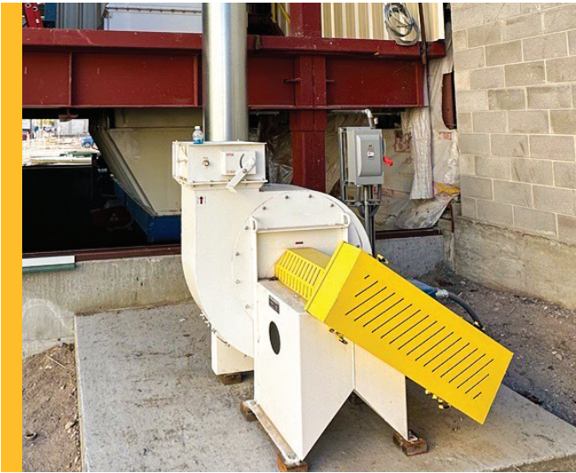
Safety Mount ISAF bearings are being installed on all air relief system fans in the manufacturing facility due to reduced maintenance and superior performance.
