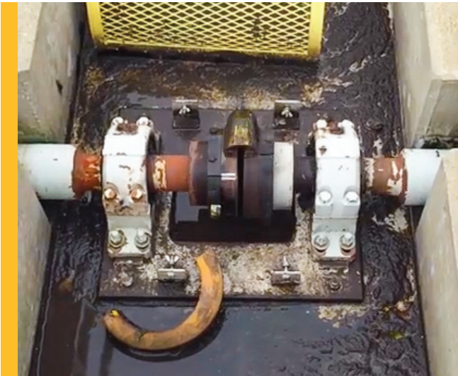
The competitive urethane couplings routinely experienced urethane bond degradation, failing to stand up to the harsh environment of the oxidation ditch.
